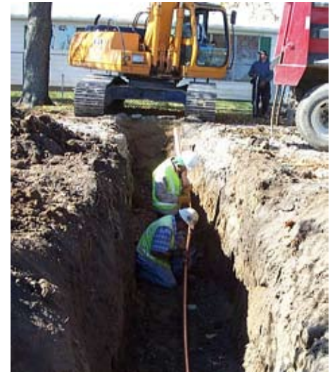
Service connection installation
