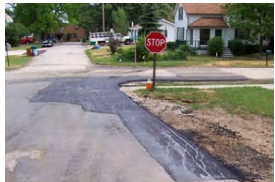
Pavement reconstruction
