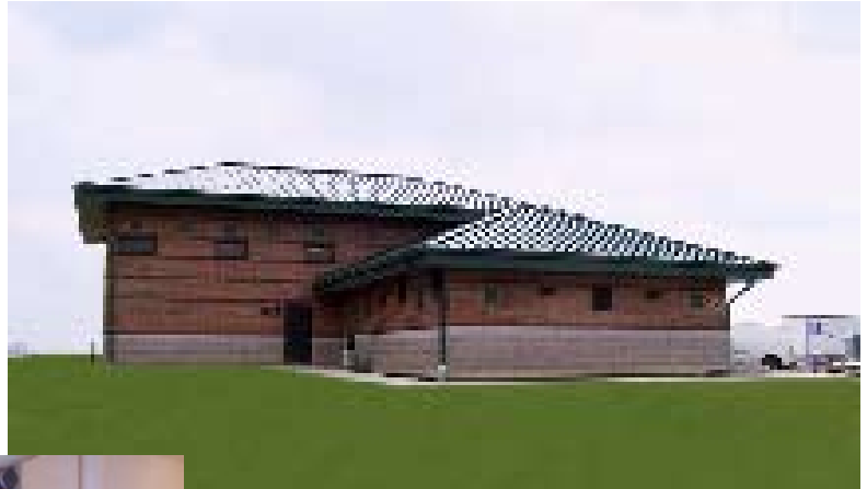
Water treatment facility
