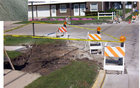
Sidewalk section under construction
