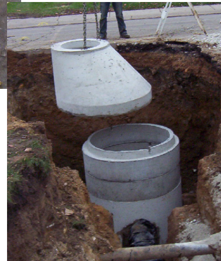
Manhole Installation
