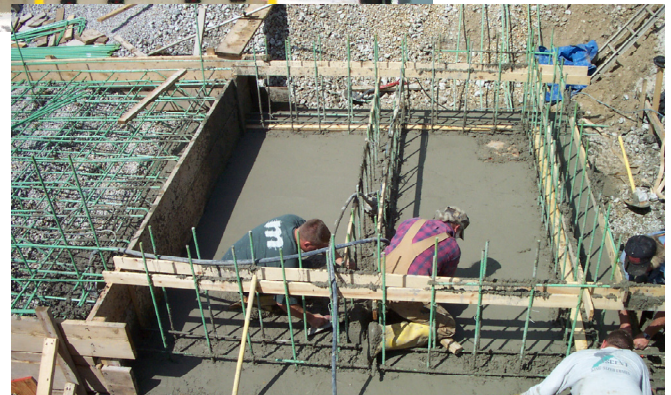
Water Treatment Facility Construction
